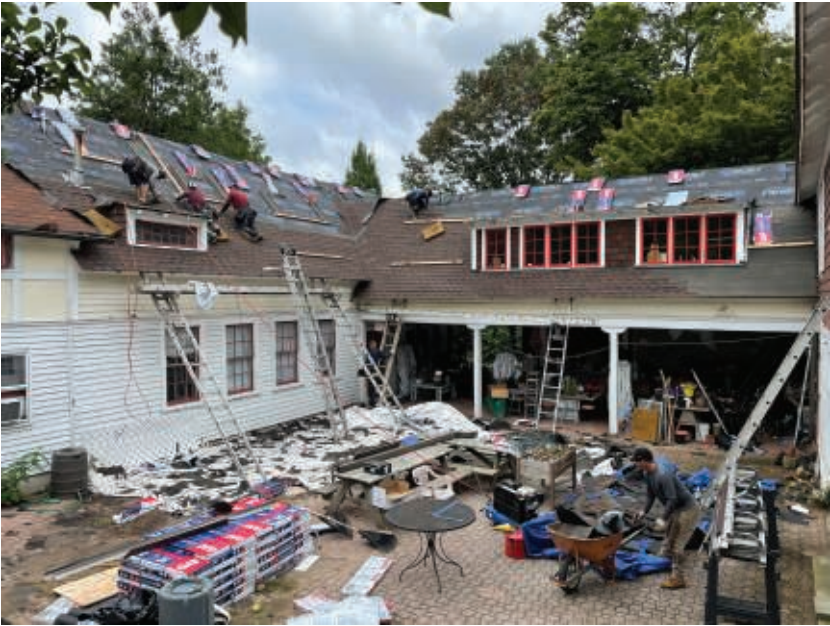
Smith Court building received a new roof and paint job.
